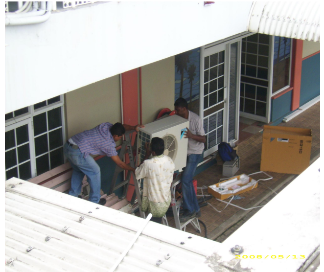
BOYS INSTALLING OUTDOOR UNIT
