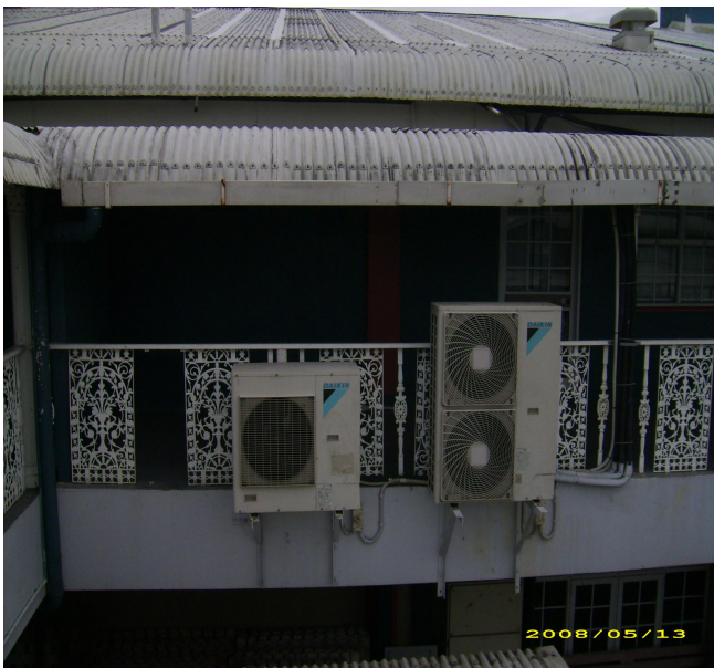
OUTDOOR UNITS INSTALLED
