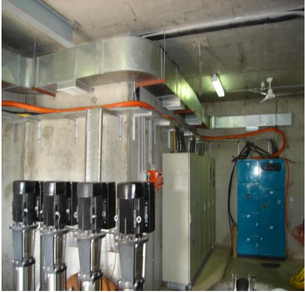
PUMP ROOM EXHAUST DUCTING INSTALLED
