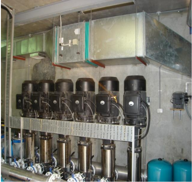
PUMP ROOM EXHAUST DUCTING INSTALLED
