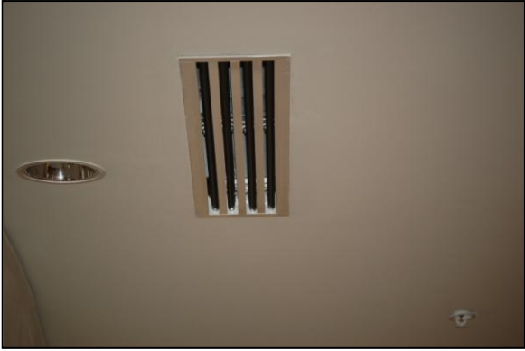
AIR CONDITIONING SUPPLY LINEAR GRILLES
