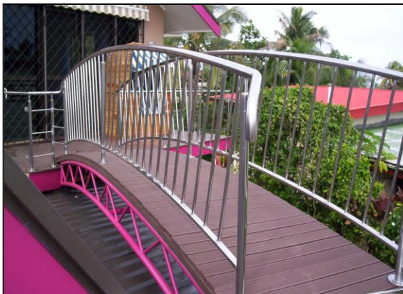
Stainless steel railing
