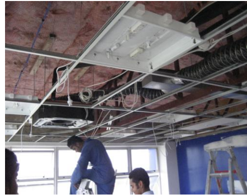
Technician installing VRV blower
