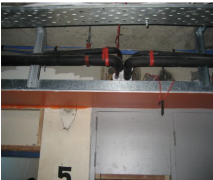
Installation of pipe works for A/C unit
