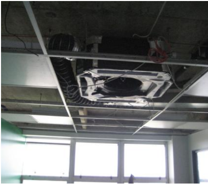
Installation of cassette system
